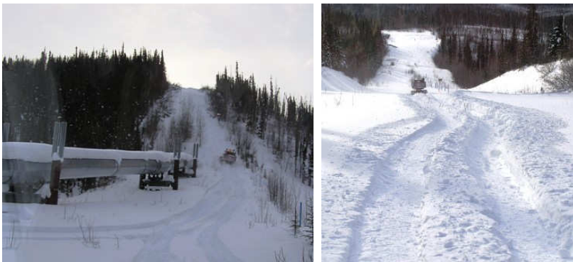
The Tucker's ability to traverse snowy terrains include that of going uphill along the pipeline (left) as well as going downhill (right).
