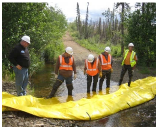
Team members looking at the dam used to contain & retrieve spilled oil.
